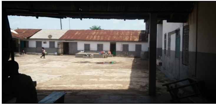
Figure 3. AgyaAhyiaAsiedu's House. Source: Field Data, March 25, 2017.
